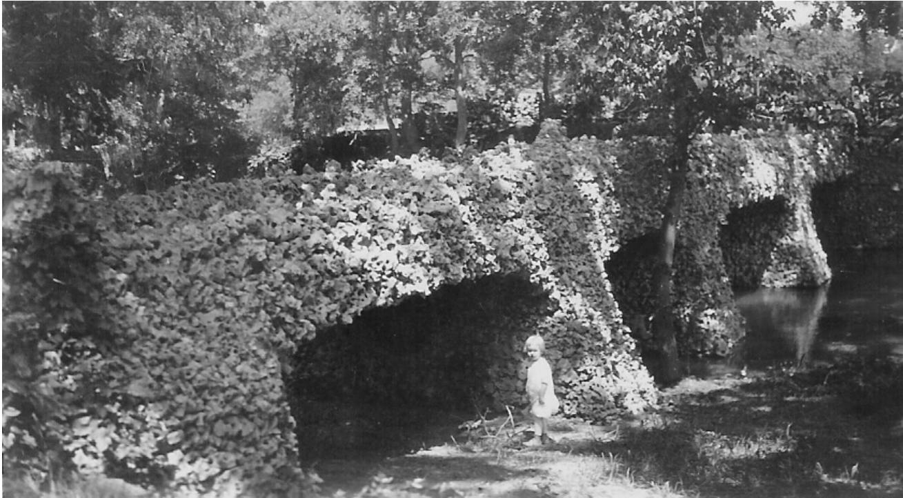
Figure 14. Madarasz Park bridge
