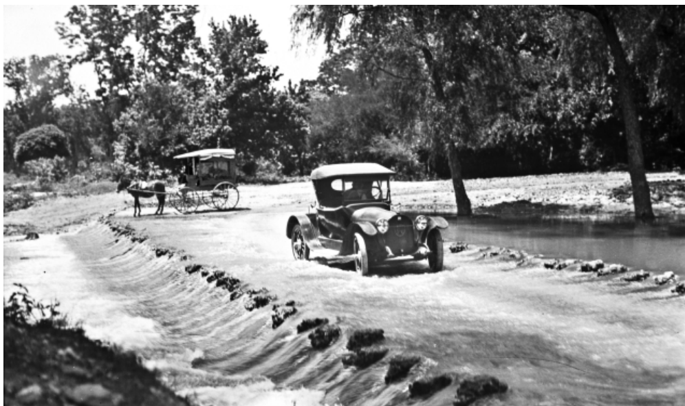
Figure 19. Low water crossing
